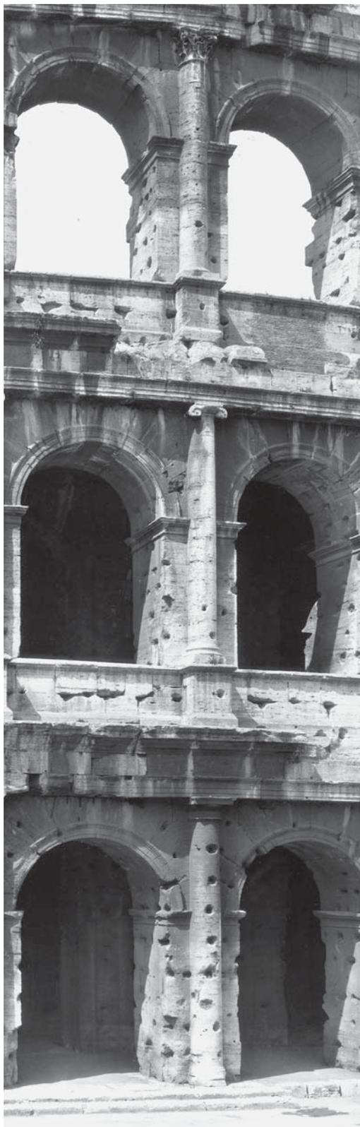
7.80 m, equal to 26 and 1/4 Roman feet, corresponding to an 8 and 3/4 module. This order appears less graceful than the Tuscan one; however, the feeling this proportion inspires is partially mitigated by the fact that it rests on a pedestal and so, by and large, it provides a balanced ratio.
