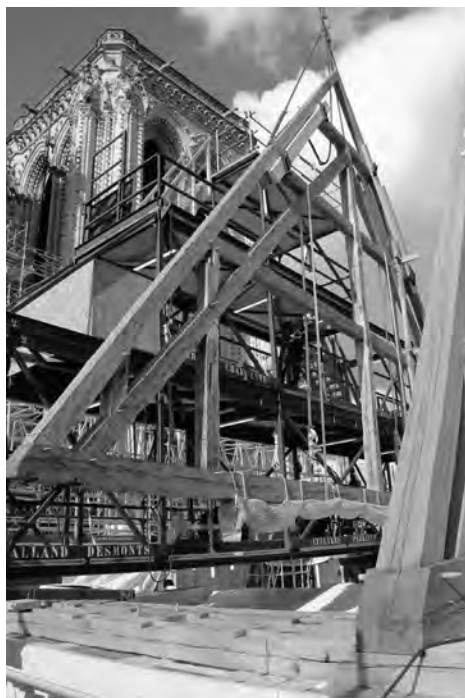
Fig. 4. Assembly of the oak timbers for the forêt in Notre-Dame, in November 2023 ( https://rebatirnotredamedeparis.fr/ ).
