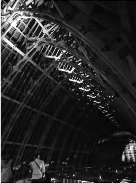
Fig. 3. Deneux trusses in Reims Cathedral.
