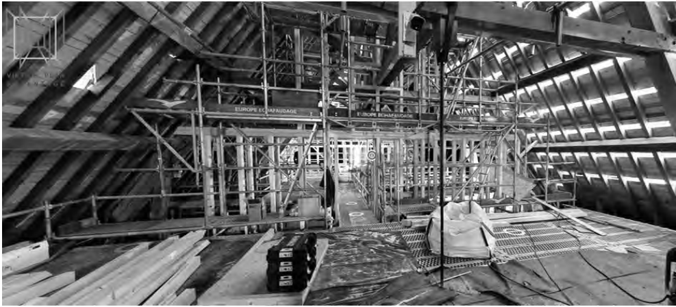
Fig. 7. Fire breaking partitions between the choir and the transept at the roof in Soissons Cathedral, November 2022 (Virtual tour in https://my.virtualplanadvantage.com/tour/chantier-de-la-cathedrale-de-soissons-charpente-08-11-22 ).
